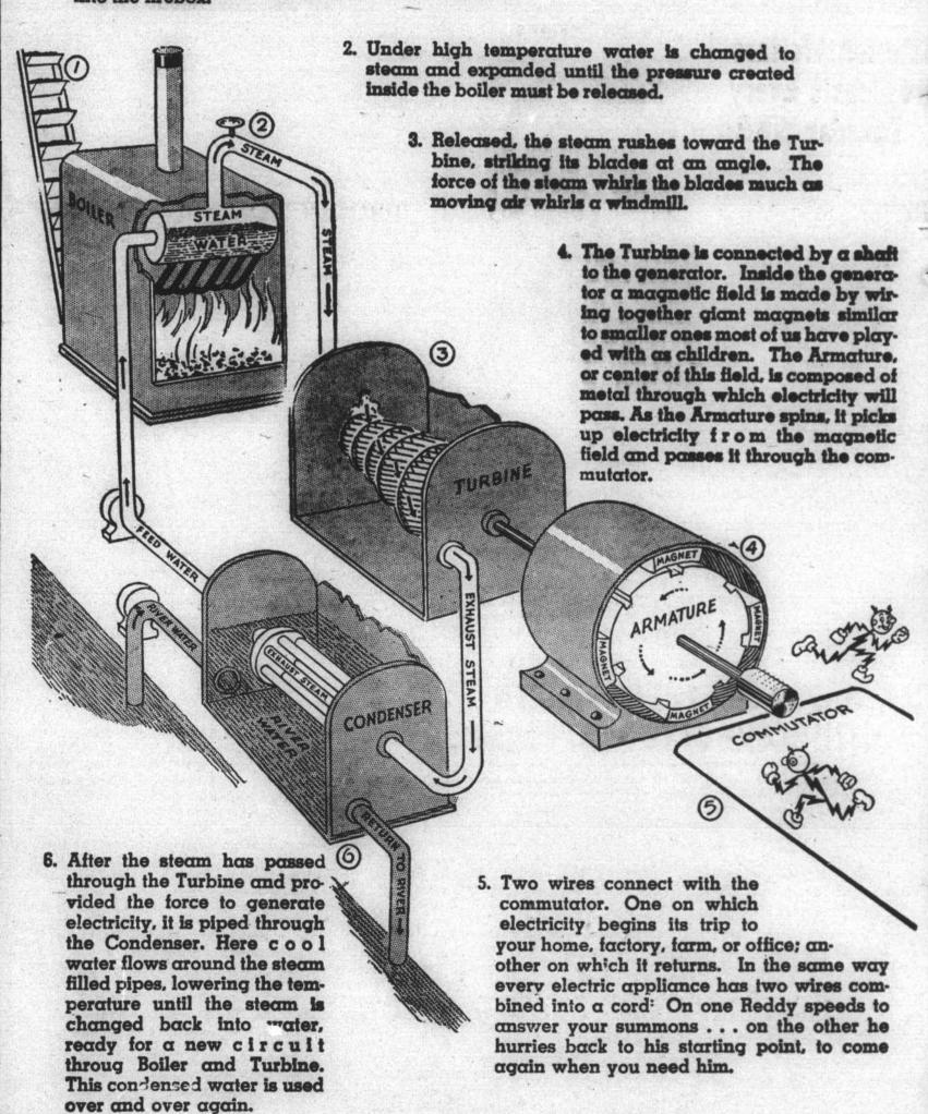
Steam plants are located on rivers in order to have a continuous flow of water to the Condenser. The cooling water returns to the river unharmed.
