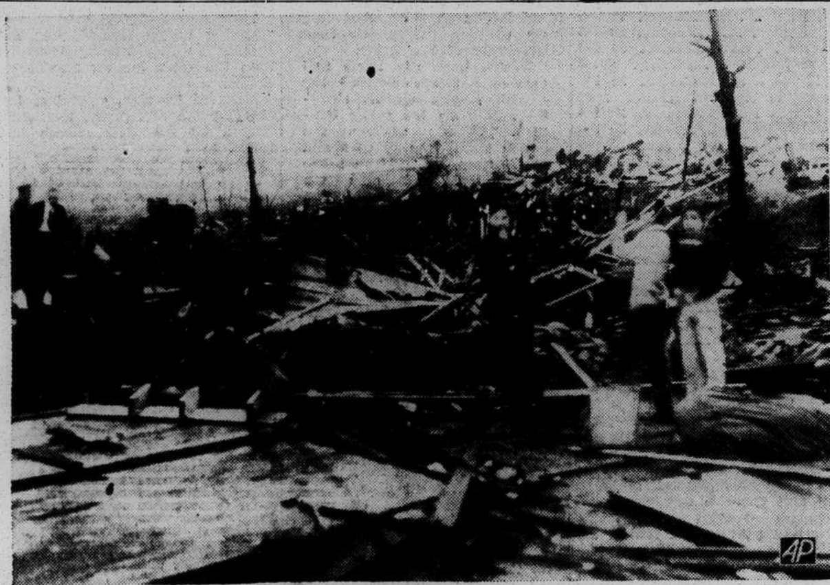
TORNADO FLATTENS HOMES IN MONTGOMERY OUTSKIRTS—Shattered, flattened homes lie in an outlying residential district at Montgomery, Ala., after a tornado swept through Feb. 12, killing at least 17 negroes and eight white persons. The main part of the city was missed by the storm's center.
