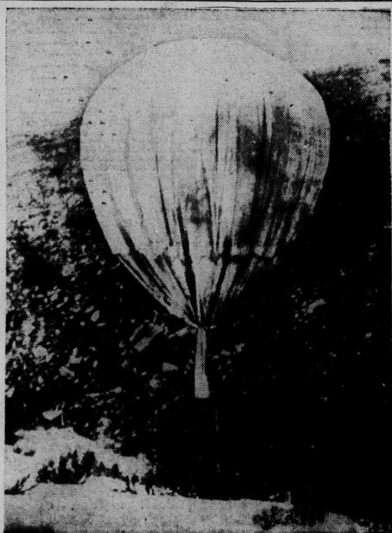
JAP BALLOON IN FLIGHT—This photograph shows a Japanese paper balloon in air over North America. They carry fire and anti-personnel bombs and are designed to destroy themselves when their explosives are dropped.—(AP Wirephoto)
