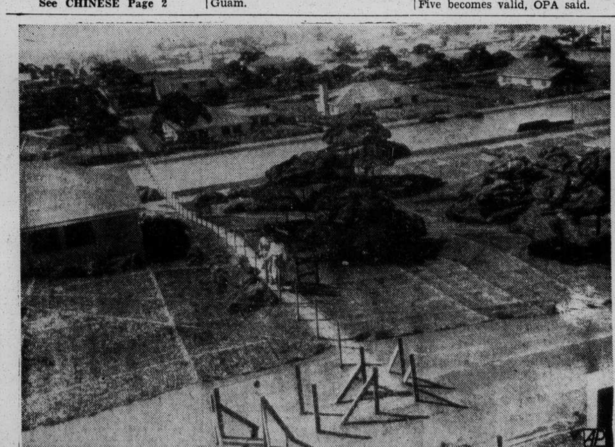
CAMOUFLAGE TOWN HIDES B-29 PLANT—Two women walk along a catwalk running through a camouflage town that was built over a B-29 plant at Seattle, Wash., to protect it from the threat of possible Jap air raids. Photograph of the project has been released now for the first time. (AP Wirephoto).
