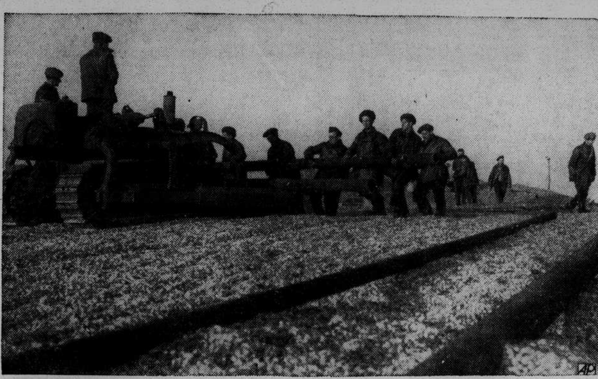
PLUTO'S SECRET REVEALED—Bulldozers carry away heavy pipelines which conveyed petrol to Pluto, submarine line from Dungeness, England, to France, which is being dismantled. Pluto supplied Allied forces during the invasion of Normandy. The secret of the line was so well kept that only now are people living in Dungeness learning of its presence.
