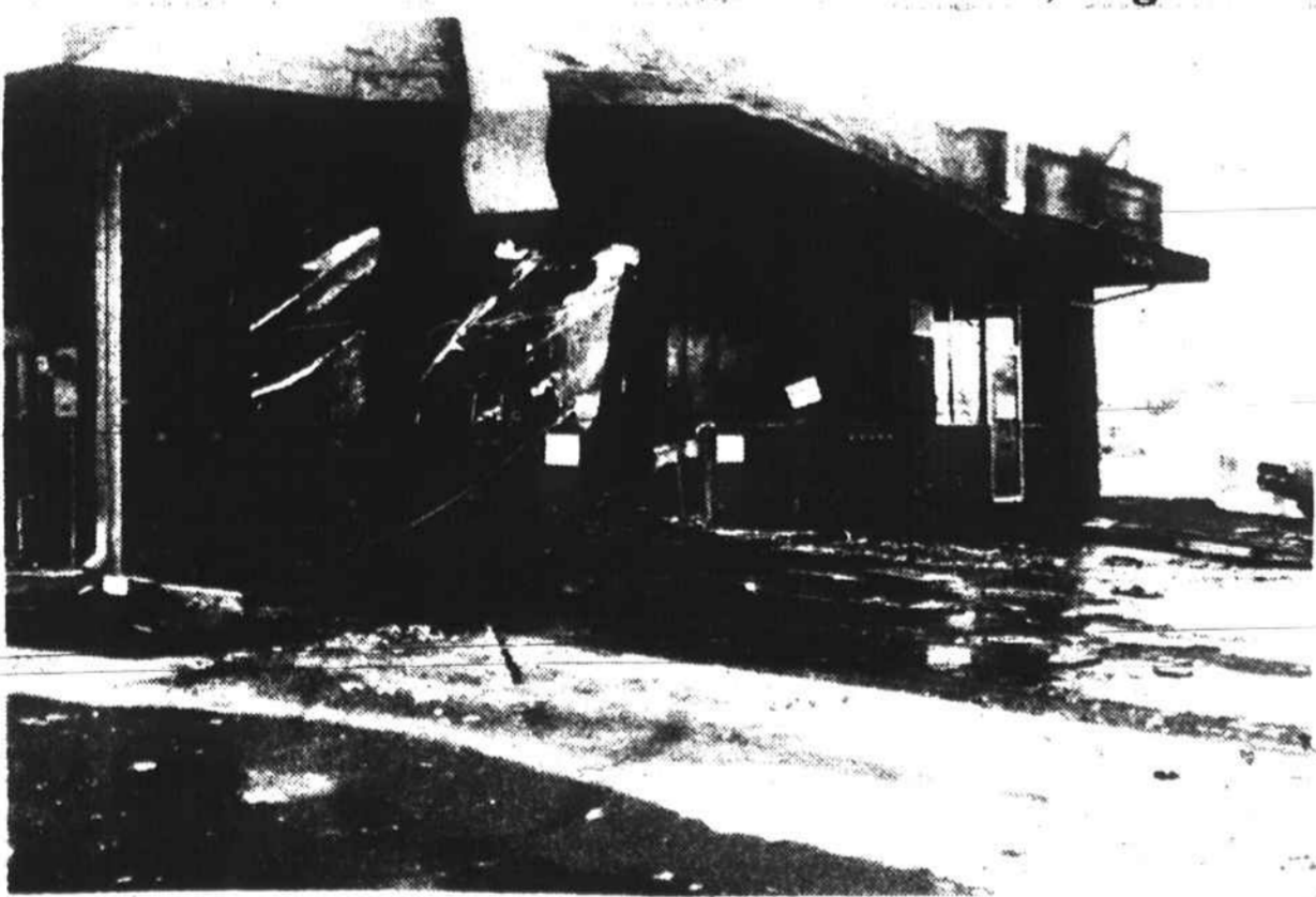
Fire ripped through this small shopping center on Old Greensboro Road. The complex is owned by Jerry Jones.
