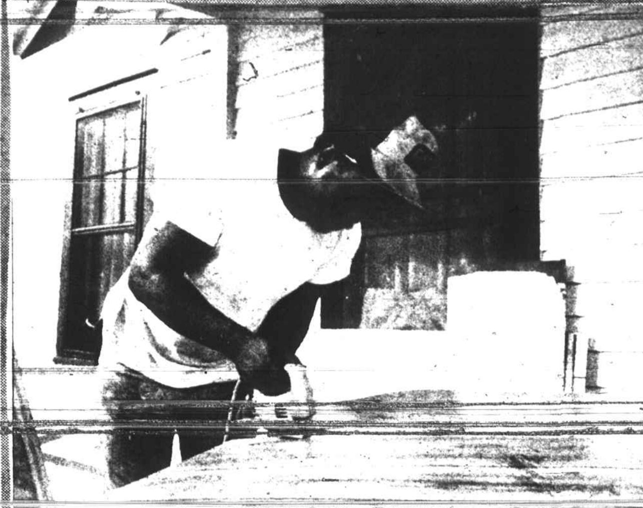
Clyde Thomas uses a skill saw to cut a piece of plywood down to size.
