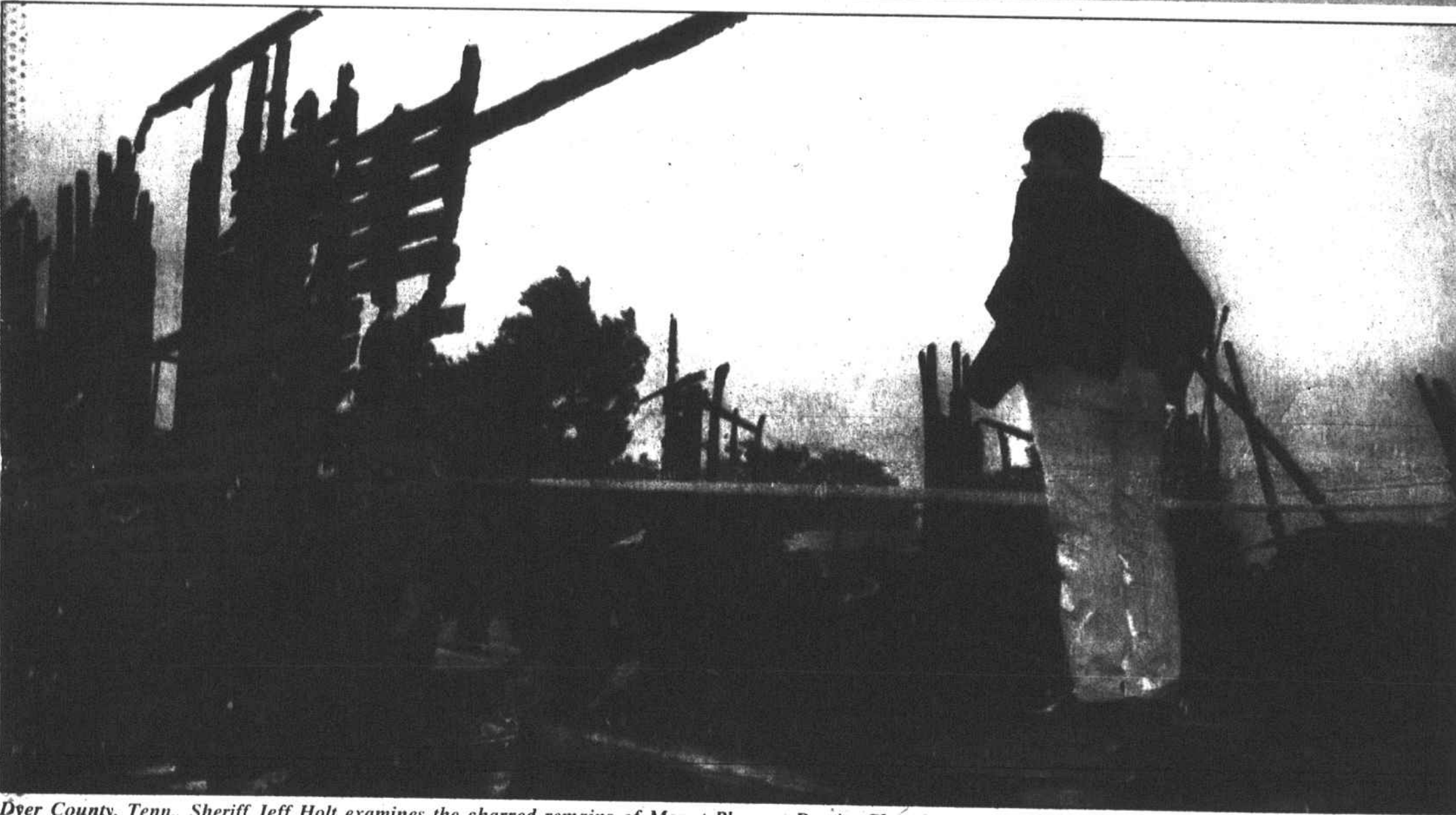
Dyer County, Tenn., Sheriff Jeff Holt examines the charred remains of Mount Pleasant Baptist Church in Tigrett, Tenn. The church was destroyed by a fire of unknown origin. Agents from Tennessee and Dyer County, the FBI, and the Bureau of Alcohol, Tobacco, and Firearms are investigating.
