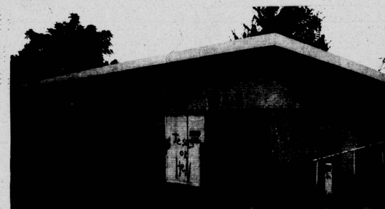
Dilapidated commercial buildings in the Old Cherry area will be torn down to build housing.
