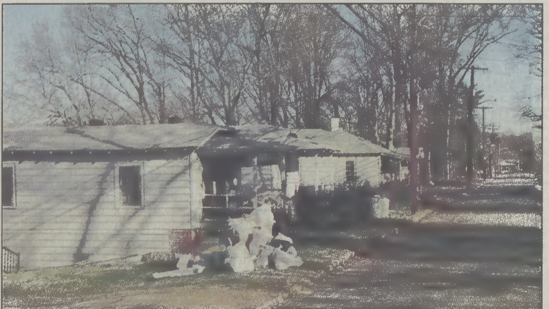
Dilapidated and unmaintained rental properties along Alder Street's park edge help give Happy Hill a negative image at its principal entrance.
