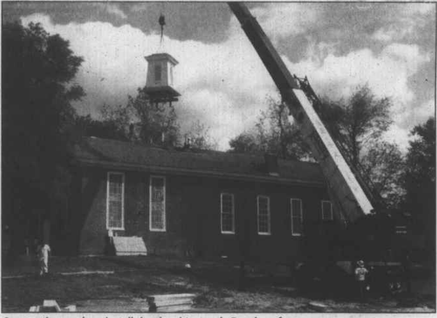
Construction workers install the church's steeple Tuesday afternoon.
