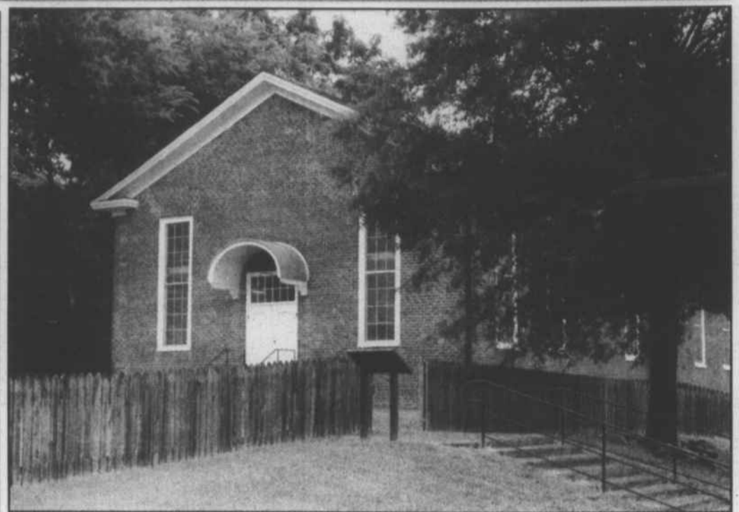
This brick St. Philips Church was constructed in 1861.
