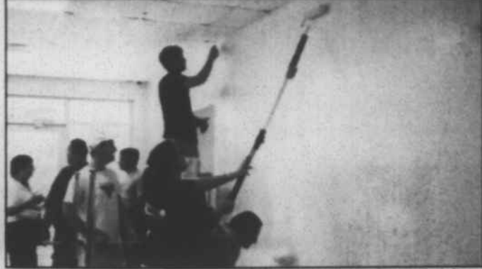
BB&T volunteers paint an interior wall.
