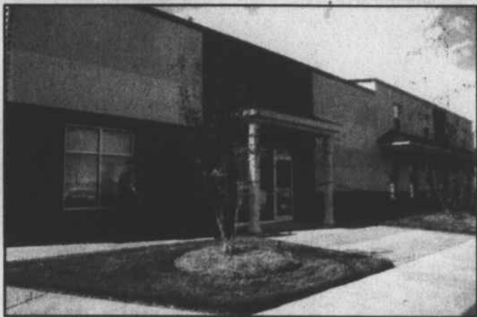
A view of the renovated facility.
