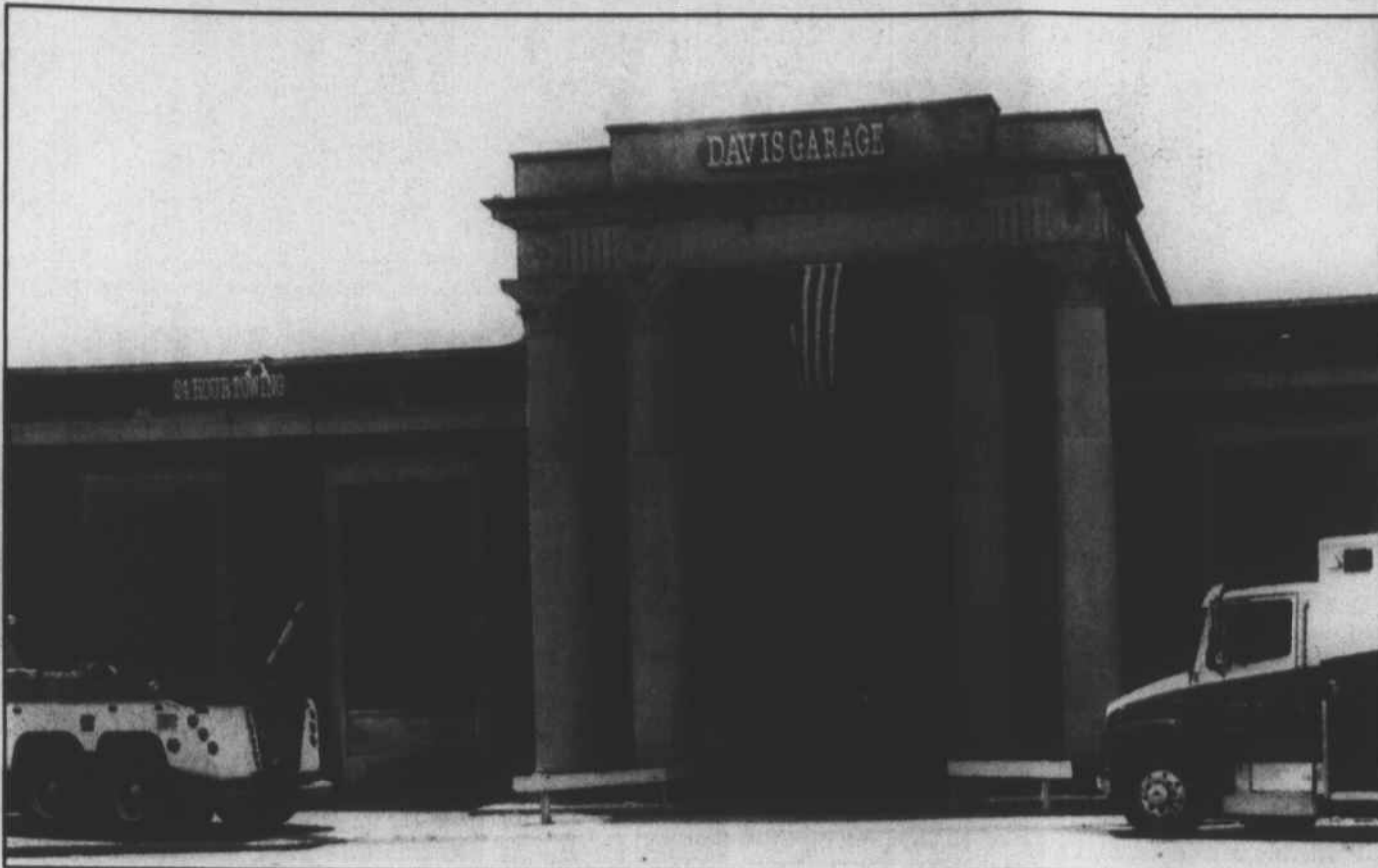
Davis Garage sits at 300 S. Martin Luther King Jr. Drive.
