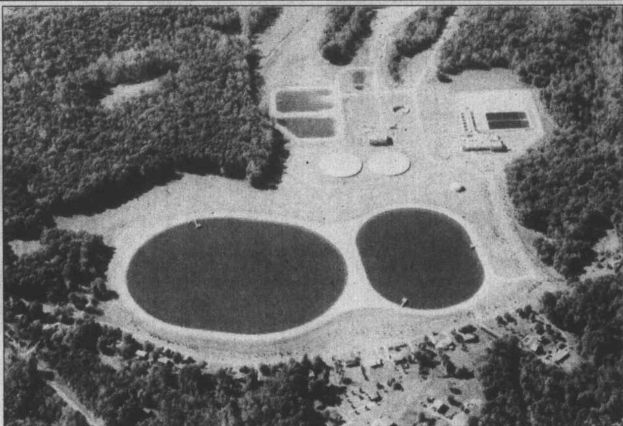
The raw water reservoirs at the Swann Water Treatment Plant hold 150 million gallons – enough to keep the plant operating for six days. This gives plant operators the ability to avoid drawing water from the Yadkin River when it is filled with sediment from a storm. This reduces the cost of running the plant.
