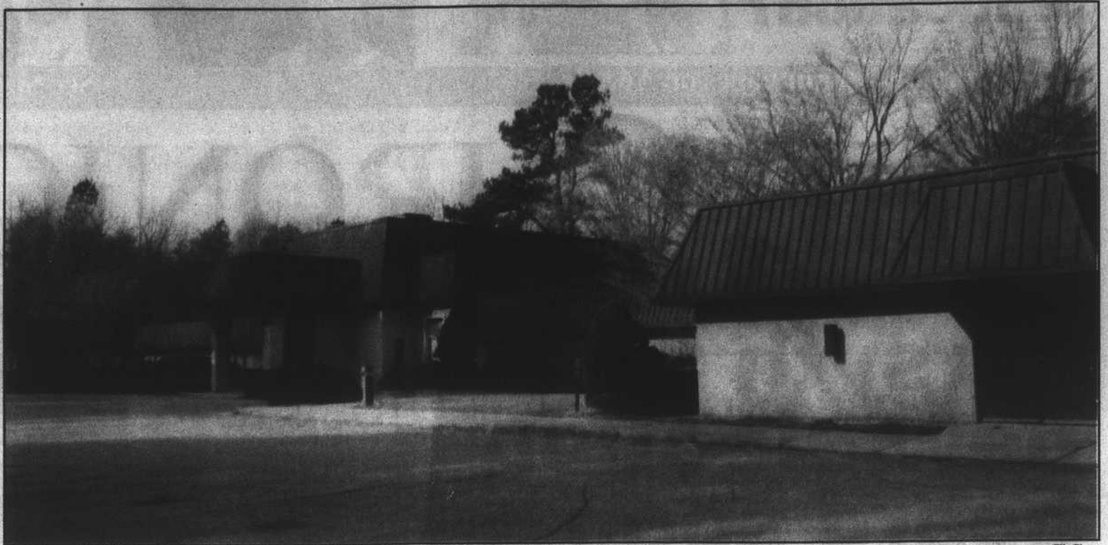
This facility on Shattalon Drive will be the new home of Addiction Recovery Care Association, Inc. (ARCA).
