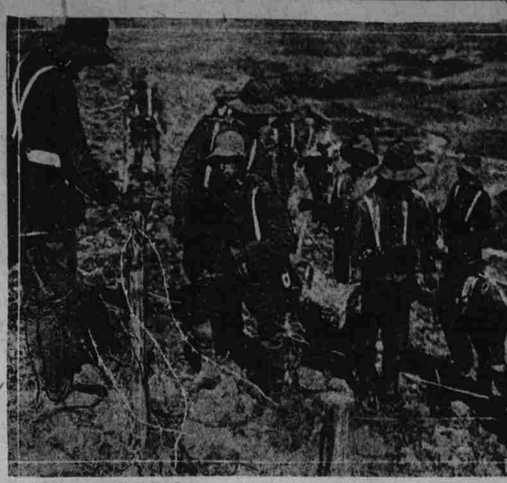
Spanish engineers erecting barbed wire entanglements "somewhere in Morocco." Scenes that recall the World war are being enacted in Morocco, Spain's last colony, where the Spanish forces are fighting an insurrection of the Moors. Barbed wire entanglements, camouflage and other kinds of war strategy are being used by the king's soldiers.
