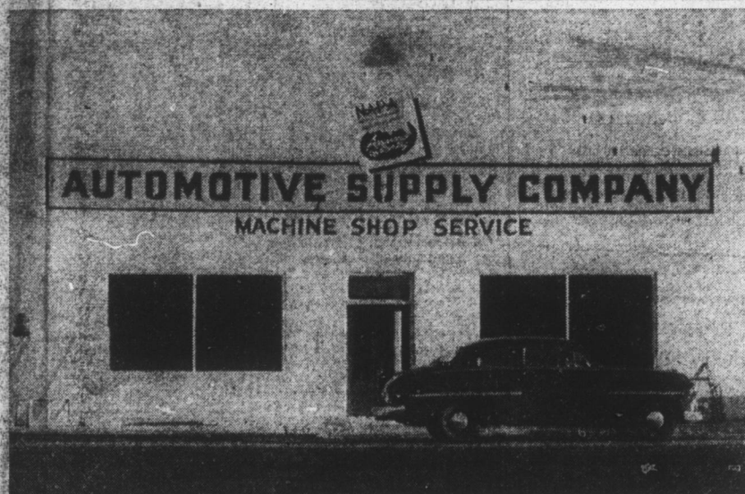
DUNN CONCERN IN NEW HOME—Pictured here is the modern new home of Automotive Supply Company of Dunn, located on North Railroad Avenue in the building which formerly served as the old Dunn Armory. The firm had a fire late last fall at their North Wilson Avenue location and moved to the new building, which has been completely renovated, improved and modernized. Automotive Supply Company, founded here in 1936, is operated by Henry Shell, Bill Barfield and Mack Hamilton, all well-known Dunn business men. The firm is a member of National Automotive Parts Association, nation-wide parts company. Mr. Shell said today that the company is planning a formal opening at a later date. (Daily Record Photo by T. M. Stewart.)
