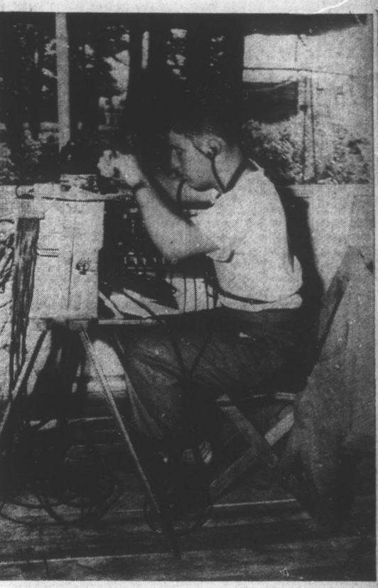
COMMUNICATIONS CENTER — Members of the 833rd Signal Operations Company, stationed at Camp Mackall, have been installing communications equipment here for use in Exercise Southern Flies. The center of the network is located behind the Dunn High School music building. Shown at the telephone switchboard here is Pvt. Milton Goretzky. (Daily Record Photo by T. M. Stewart.)
