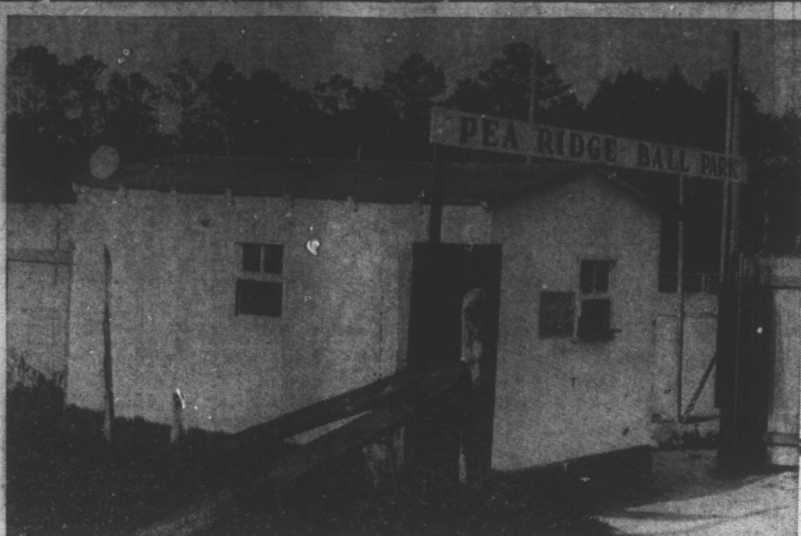
THIS VIEW OF THE OUTSIDE OF THE PEA RIDGE BALL PARK shows the entrance and ticket office and concession stand. The ball park is located in a rural section, and it was built by the people of the community who wanted to have a baseball team very much. The story of the building of the park is told in an article by a member of the community. (Daily Record photo by T. M. Stewart).
