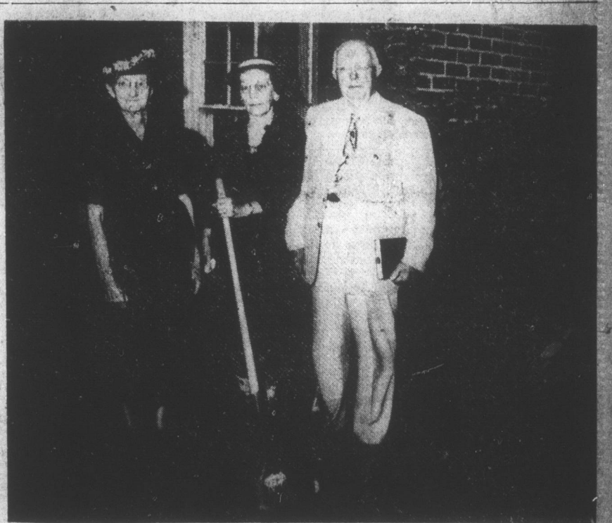
GROUND-BREAKING RITES - Mrs. R. F. Jernigan, oldest member of Hood Memorial Christian Church from standpoint of years service, is shown here with the shovel at ground-breaking rites held Sunday night marking the beginning of the new $35,000 educational building.
