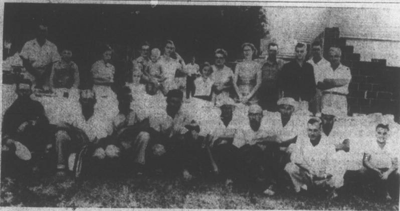
TIME OUT FOR LUNCH — Members of the Dunn Advent Christian Church are doing the work themselves on the construction of a handsome new church building here. This picture was made last Saturday during the lunch hour when the ladies spread a picnic lunch for the workmen. Left to right are, kneeling: J. E. Fields, Albert Sutton, Leslie Blackmon, Dan Woodall, Woodrow Whitman, Rev. Lee Stancil, Lee Massengill, Clarence Raynor, Tom Woodall and J. W. Johnson; standing, Monroe Allen, Kirby Johnson, Ruth Fields, Mrs. Harold Hodges, Mrs. Janette Stewart, James Stephenson, Joyce Stancil, Mrs. Myrtle Strickland, Mrs. Lee Stancil, Chester Stanley, Donald Hudson, Rev. J. W. Smith and J. V. Stephenson. The group will be at work again tomorrow. (Daily Record Photo.)
