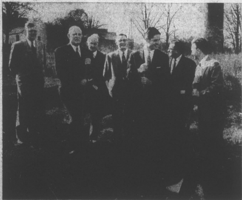
BREAKING THE GROUND — Shoveling the first dirt to break the ground for the new Branch Sunday School building here yesterday were: Mack M. Jernigan, left, chairman of the building committee, Rev. Earl Davis, Farthing, pastor, and Rev. W. L. Davenport, the first pastor. Looking on behind, left to right are Rev. Ernest F. Russell, Lonnie R. Norris, W. E. (Bill) Cobb and L. L. (Leck) Coats. (Daily Record Photo.)
