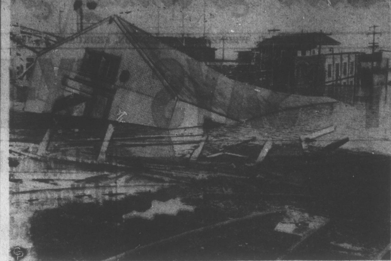
A CHEMICAL PLANT BUILDING ON THE Detroit River, near Windsor, Ontario, is partly submerged in the river as a result of the collapse of an abandoned old salt mine. Two large warehouses sank into the ground and others tilted when the underground mine caved in. Six hundred workers at Canadian Industries, Ltd., and the Canadian Salt Company ran out when the buildings shook and then began to sink. Many areas of Windsor and southwest Detroit are honeycombed with abandoned salt mines. (International Soundphoto)
