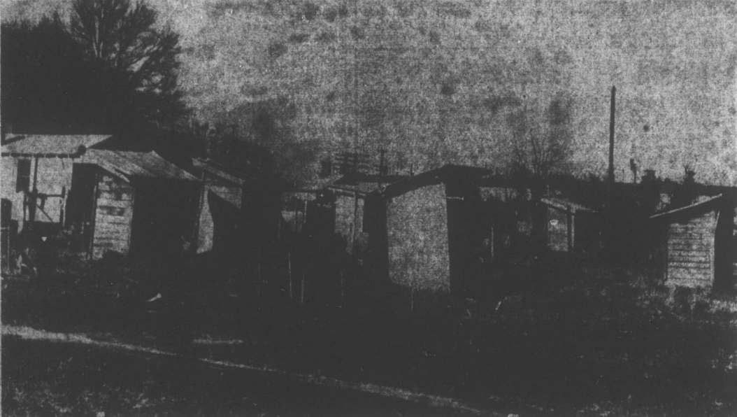
YES, THIS IS IN DUNN — You may not believe this, but the above picture was taken within the Dunn City limits. It is on Granville Street, between King and Layton Avenue. A town ordinance requires that all homes within 200 feet of a sewer line must lap on and destroy outside toilets. All of the above toilets are within 200 yards of a sewer line, yet some 12 toilets are still in use in this area. A six inch sewer line has been run within 200 feet
