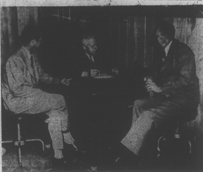
FRIENDLY POW WOW — These familiar faces at the Bank of Lillington are having a conference, as they do most any day, but the meeting is new, the bank's new building which will be displayed to the public for the first time on Thursday from 7 to 9:30 p. m. The men are John W. Spears, center, cashier; and his assistant cashier, Roger Mann, left; and J. Grady Johnson, right.
