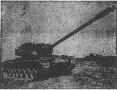
THE HEAVIEST and most powerfully armed of U.S. tanks, the long-secret T-43, is show first time at Newark, Delaware, where for three years it has been in production. The arm signed by Army and private plant engineers, mounts a 120 mm. cannon and .50 and .30 calibe
