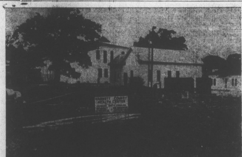
HEALTH CENTER RISES Foundations for the new Harnett County Health Center have been erected and walls of the new building are rising rapidly. This photograph shows where the center will be located on the Northeast side of the courthouse square. Small frame building at right is the county library. Once the center is finished, library will occupy quarters in the agriculture building which the present health department staff will vacate for the new center. Tree adds to attractiveness of site. (Daily Record Photo by T. M. Stewart)
