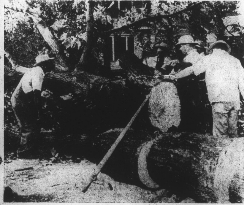
REMOVING TREE - City workmen are pictured above as they sawed a large oak tree into small blocks to move it off the street at the corner of S. Wilson Avenue and Cumberland Street. The tree fell on a car parked on S. Wilson Avenue. City Manager A. B. Uzzle said today that it would take at least two days to clear trees off the streets here. (Daily Record Photo.)
