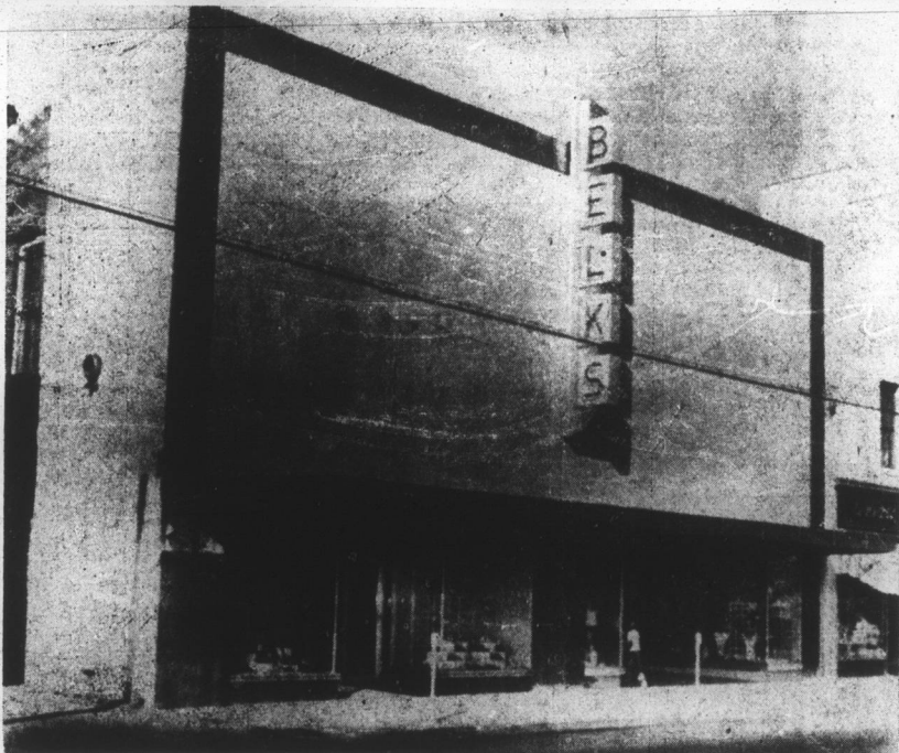
BELK'S NEW FRONT - Pictured here is the beautiful new front of Belk's Department Store in Dunn, added at a cost of several thousand dollars. The big department store has also made a number of other improvements, including the installation of a modern elevator. Marvin Raynor is manager of Belk's, one of the largest department stores in this section of the State. (Daily Record Photo.)
