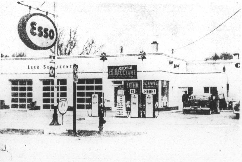
SKINNY'S ESSO HAS NEW HOME—Skinny's Esso Station at the corner of Broad and Fayetteville in Dunn has been completely remodeled. In fact, the old station was torn down and this beautiful and modern new structure was erected in its place. It is one of the prettiest stations in this section. The station is operated by Howard (Skinny) Ennis. (Daily Record Photo.)
