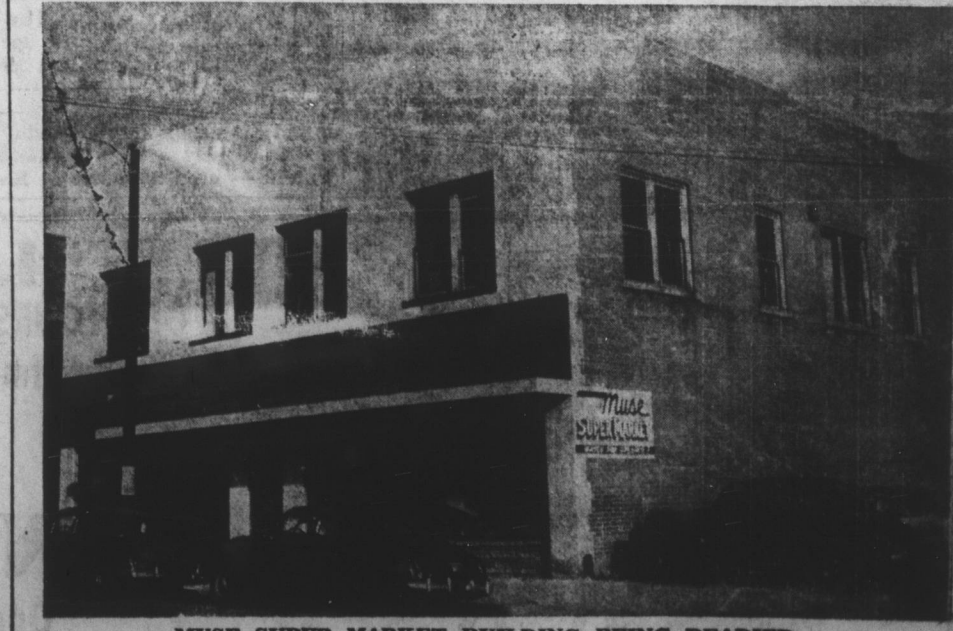
MUSE SUPER MARKET BUILDING BEING READED
