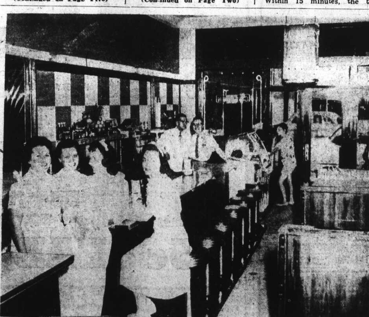
NEW RESTAURANT OPENS — A downtown restaurant featuring drive-in service and an unusual doughnut-making machine opened its doors today. Owner and manager is West-Coates, who formerly ran the E&W Restaurant on the same site. Called the Dunn Restaurant, its
