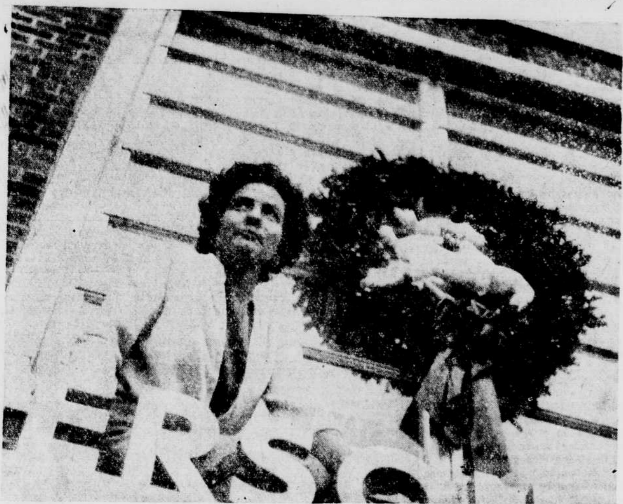
RAMPANT REINDEER — Giant wreath enclosing a hard-charging reindeer is part of decorative scheme at Anderson Arms apartment house on West Broad Street. Reindeer is on second floor and Frances Surles, taking a look down avenue where everybody else was decorating, too, had to
