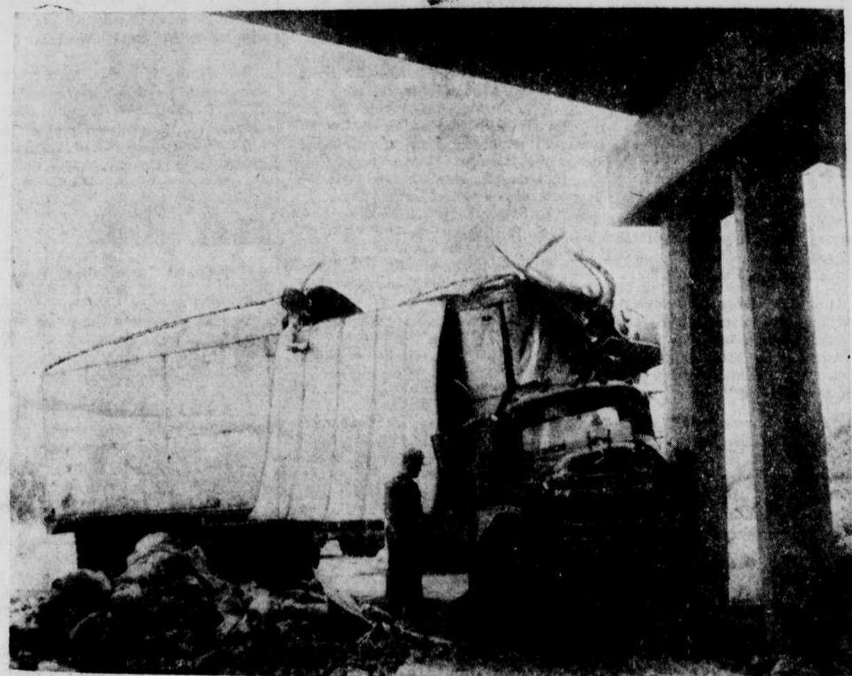
TRUCK HITS BRIDGE — Rookie Patrolman Charles W. Rogers surveys crumpled trailer-truck which crashed into a bridge spanning new Interstate 95 on the Harnett-Cumberland line. The out-of-state driver, hauling big load of potatoes, crashed through a barricade marking unopened part of the highway, swerved across road and hit bridge stanchions. He suffered minor injuries. The company suffered about a $10,000 load. (Record Photo by Ted Crail.)
