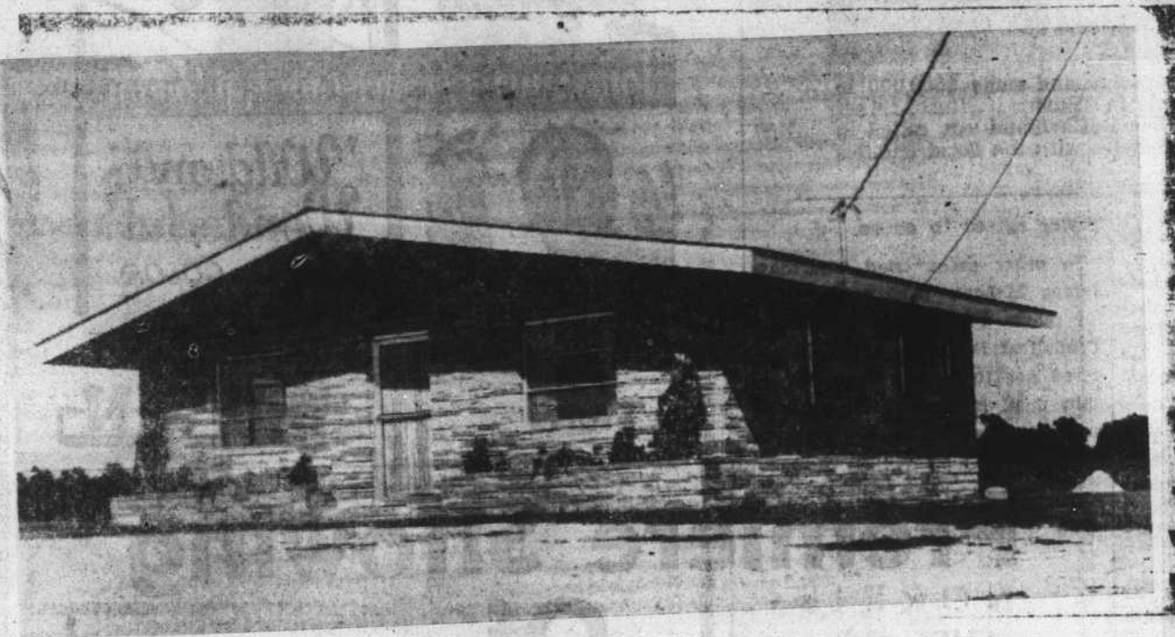
MODERN NEW OFFICE was recently constructed of Tennessee split marble. All construction work was done by J. P. Smith, co-owner, with the assistance of Devotional Garden's maintenance department. The new office is complete with a family room.
