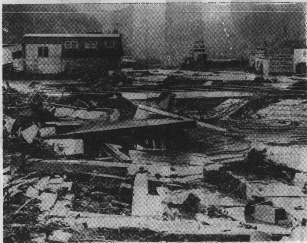
SCENE OF DESTRUCTION — This is the flood devastation in the central part of Klamath, Calif. Photo was made from the main thoroughfare, Highway 161.
