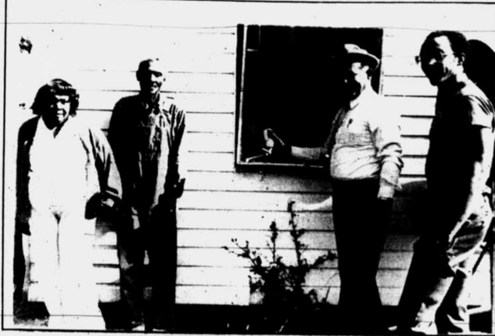
Mr. and Mrs. Charlie Gregory, left, watch David Waymer of the Agricultural Extension Service, and Kenny Garrett of 4H weatherize their home. (Photo By Teresa Simmons)
