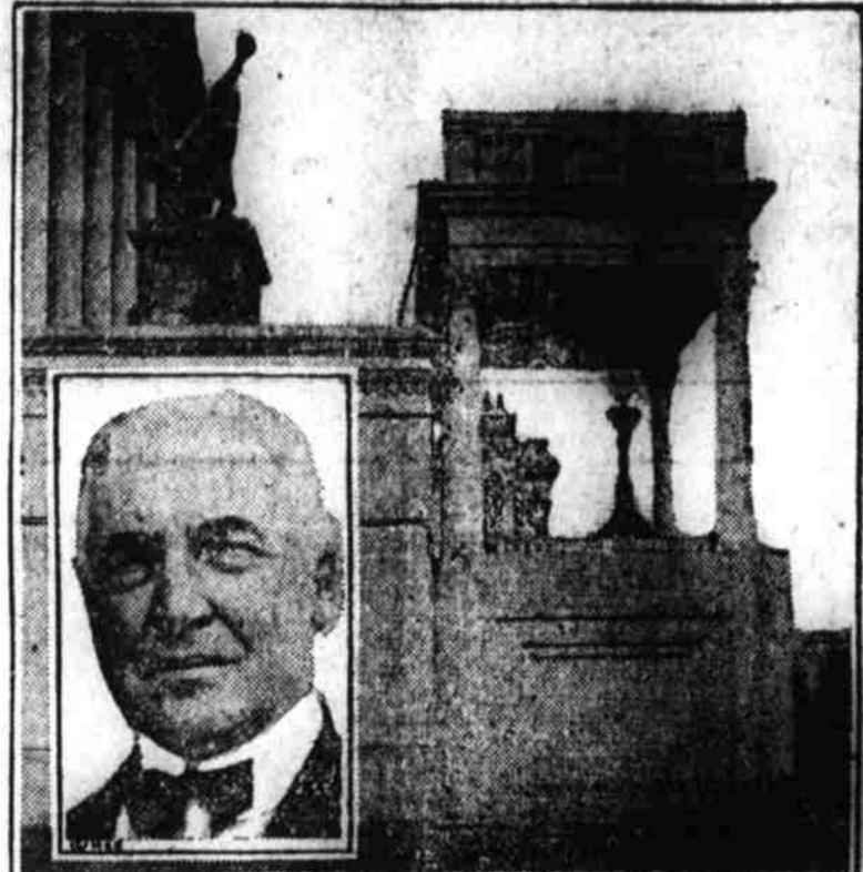
This is the completed inaugural stand where President Harding took the oath, today.
