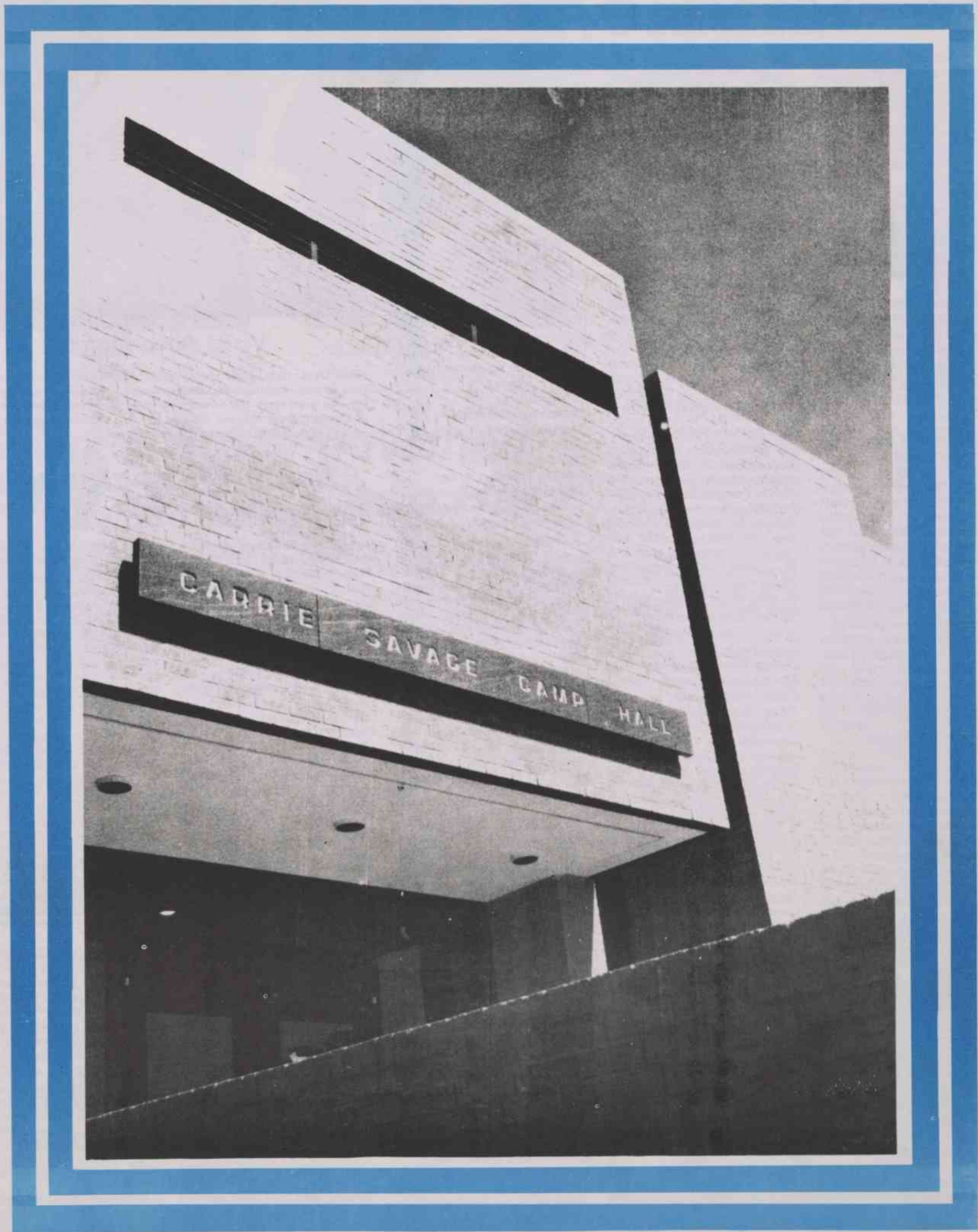
Carrie Savage Camp Hall, Chowan's new science-engineering facility, will be dedicated May 19, 1974, in conjunction with the college's 126th Commencement Exercises. The structure is named in honor of a beloved student who graduated in 1881 while her father, the Reverend Robert R. Savage, served as Chairman of the Board of Trustees.
