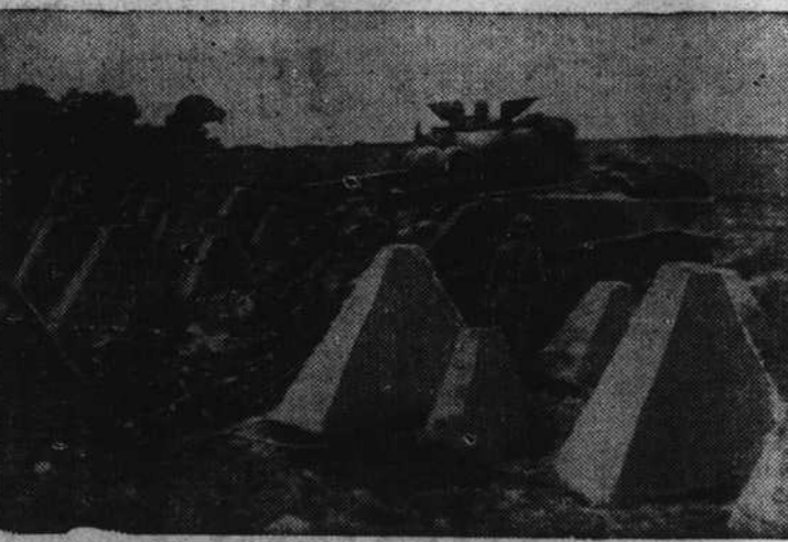
Following a path blasted by U. S. army engineers, an American tank passes through a belt of concrete and steel dragons teeth obstacles in the Siegfried line near Aachen.
