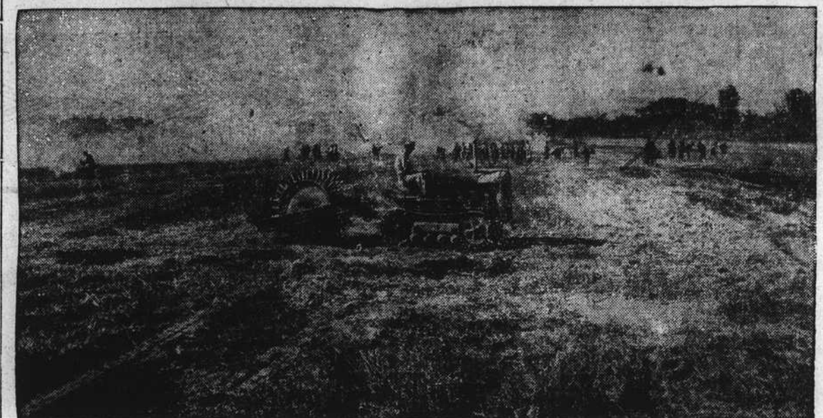
A U. S. soldier operates an American tractor and sheepsfoot roller, smoothing filled ditches on a field being prepared as an 0-47 strip in China. Coolies are cutting burning grass in the background. (U. S. Signal Corps Photo)
