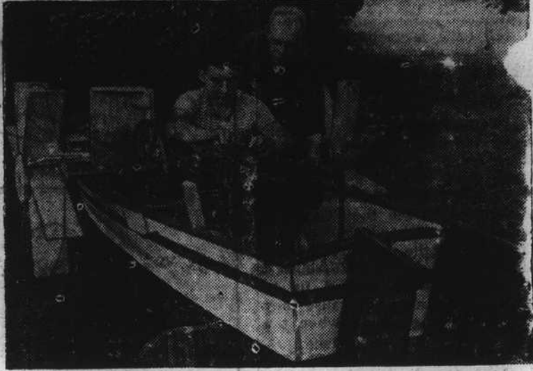
George A. Bucher gives his son, David, a helping hand to complete the latter's idea of building a sidewheeler at their home at Lake Mohawk, N. J. The boat is 14 feet long and driven by a two-horsepower gasoline engine, connected by a belt with a shaft on which are mounted two 304-inch paddle wheels.
