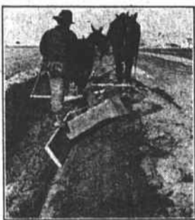
Using "A" scraper in building head ditches.
