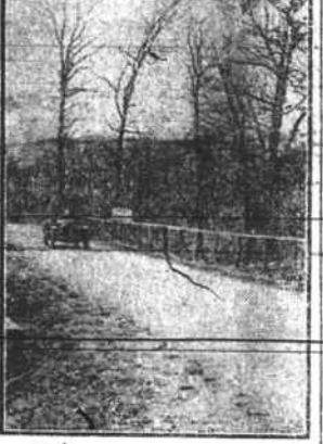
A STATE HIGHWAY IN MARYLAND.
