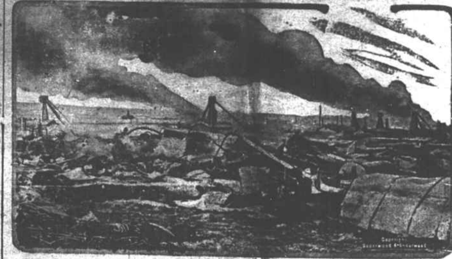
When the Russians captured part of Galicia, with the oil wells at Boryslav, their oil supply was at such a low state that they drew on the wells to their utmost capacity. The Austrians, cut off completely from their main supply of oil, fought desperately to drive the Russians out. They succeeded in doing only to find, on their return to Boryslav, the oil wells on fire. This remarkable picture of the progress of the war was made shortly after they had been fired by the retreating Russians. The boring towers in the foreground were blown up by the czar's army.
