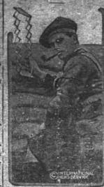
This folding periscope for use in the trenches is easily portable and is use largely by the British.
