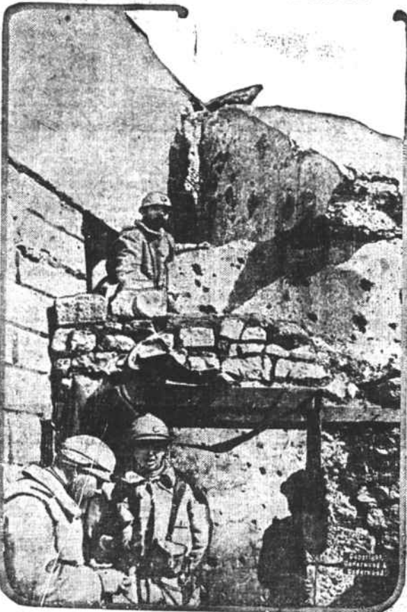
Massive block of concrete, part of Fort Douaumont's defensive wall, destroyed by explosion of mine. Fort Douaumont is the pawn of the Verdun front. It has changed hands several times and is now held by the Germans. The slaughter of troops at this point is frightful.
