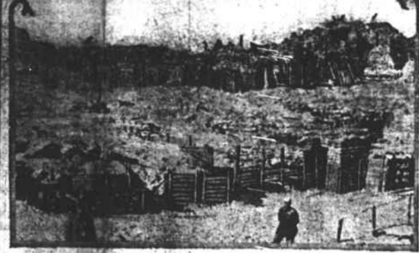
Photograph shows the remarkable construction of German trenches on the sands of a beach on the extreme southeast of Flanders. Boomproof shelters have also been built out of timber work, and sand and sand bags.
